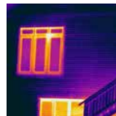
Thermal image of a home with ICFs.
