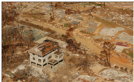
ICF home left standing and surrounded by rubble in the aftermath of Hurricane Katrina. Source: Insulating Concrete Blocks Association, "ICFs Stand Up to Storms"
