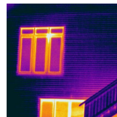
Thermal image of a home with ICFs.
